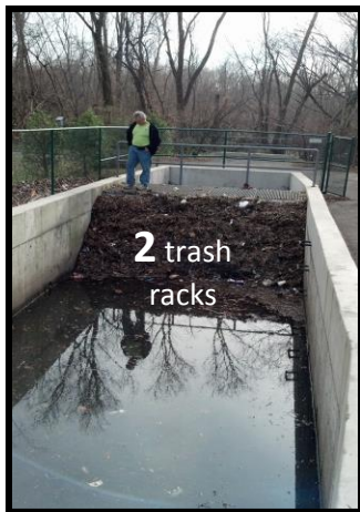
Trash rack in the Murfree Springs Wetlands
