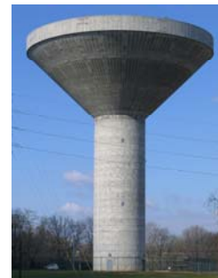
Jones Boulevard Tank
